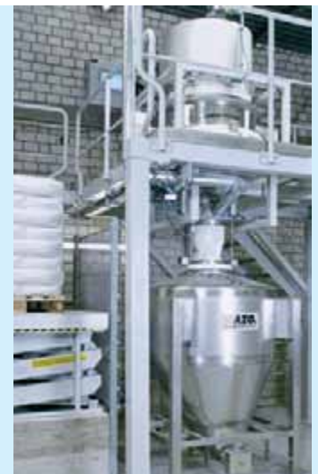
Conversion of sacks into AZO DOSITAINERS®
